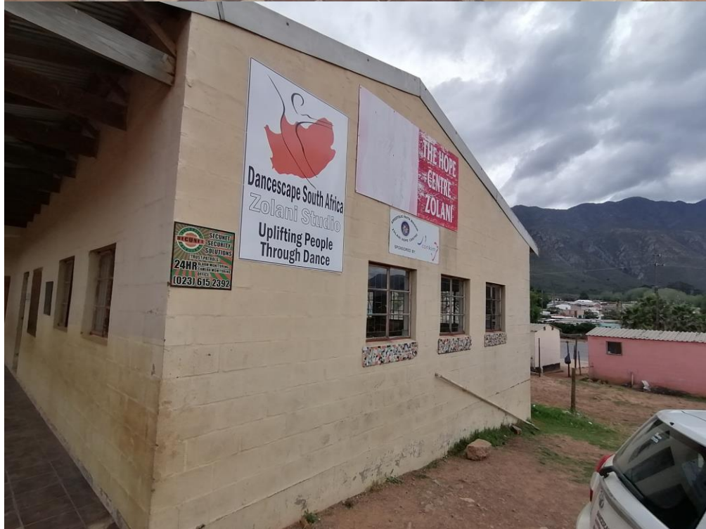
Above: The Zolani Hope Centre before the painting work began
