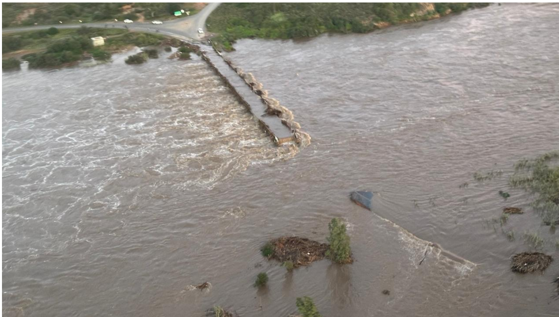
Above: Floods cause a lot of damage by washing the McGregor bridge away.
